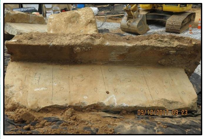
Concrete demolition was performed after sample results indicated some chemical contamination was present in portions of the concrete retaining wall and footers.
