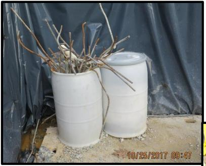
Once the concrete and rebar are separated and broken down to the correct size, they are loaded into drums and then transported to the Federal Property for storage, until shipped to an appropriate disposal facility.
