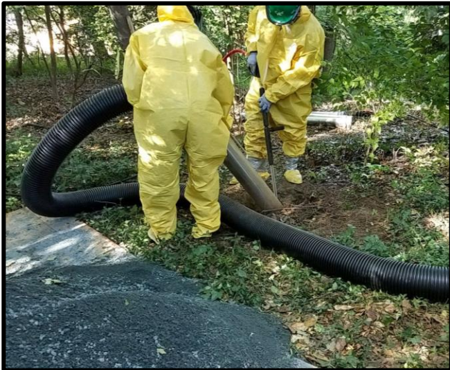
Hydro-excavating to minimize damage to tree roots in certain locations
