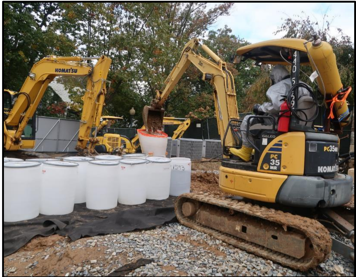
Crew working in Level B gear using a mini-excavator to load soil into drums
