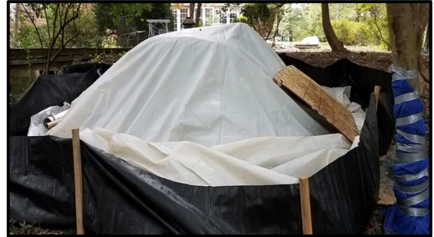
Staged clean back fill soil covered for inclement weather
