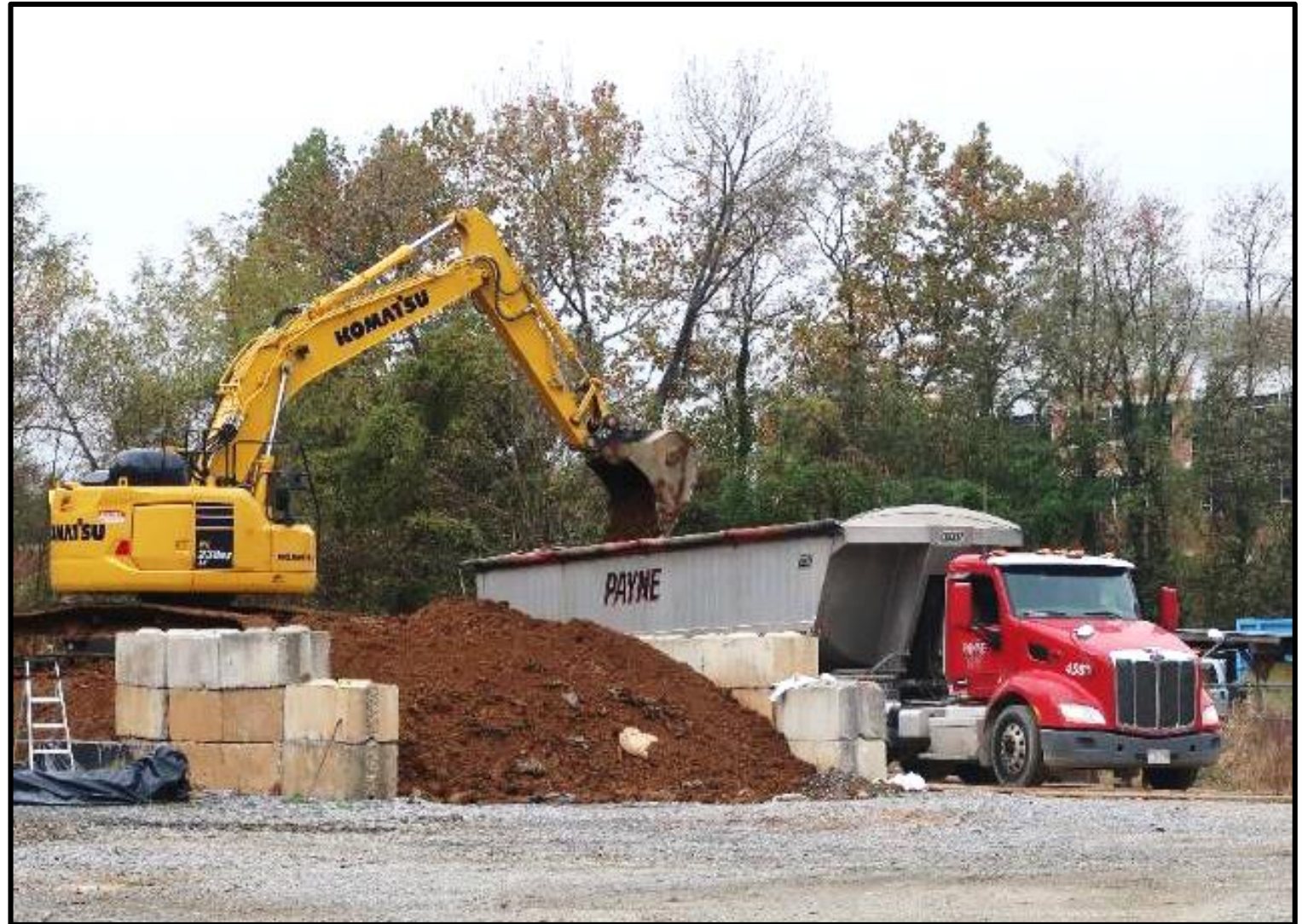
Loading a truck with soil for the Subtitle D landfill.
