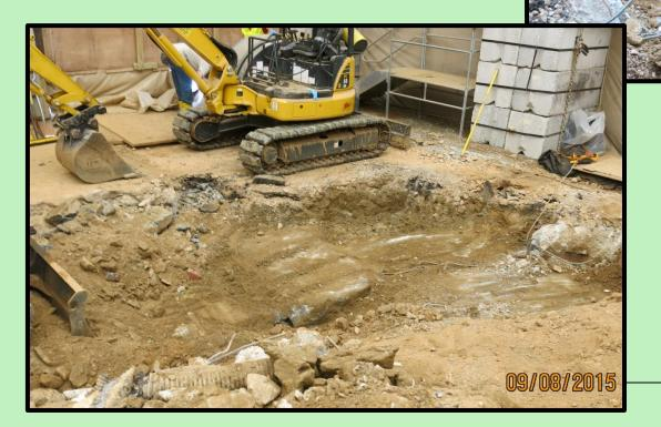
The crews are excavating under the former basement floor area to saprolite.
