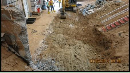
The crews began demolishing a nine foot wide section of the back basement floor, as well as the adjacent remaining section of the footer from the basement wall. This is the only section of the basement floor that will be demolished under Tent 2.
