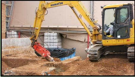
After removing the concrete surrounding the crawlspace area, the crews investigated and removed the soil inside. Due to recovering only small amounts of broken American University Experiment Station (AUES)-related glassware and no signs of stained soil in the crawlspace, the effort went quickly.
