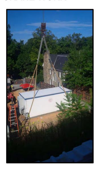
In early August, the crane was repositioned at the site to assist in the removal of the remaining heavy equipment and the large Chemical **Agent Filtration** Systems located near the back of the property.
