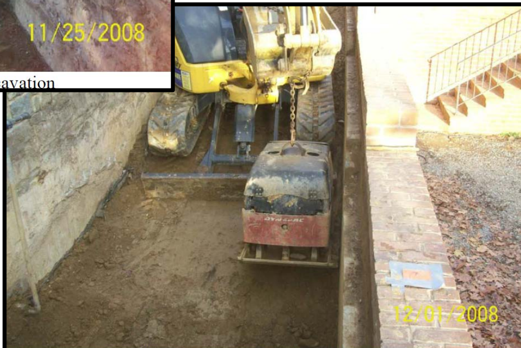
Figure D-202 Test Pit 67 backfill complete
