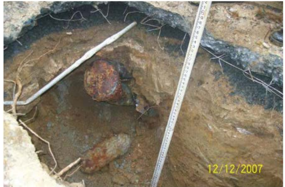
Livens projectile found at 5 ft bgs (subsequently fell to floor of excavation).
