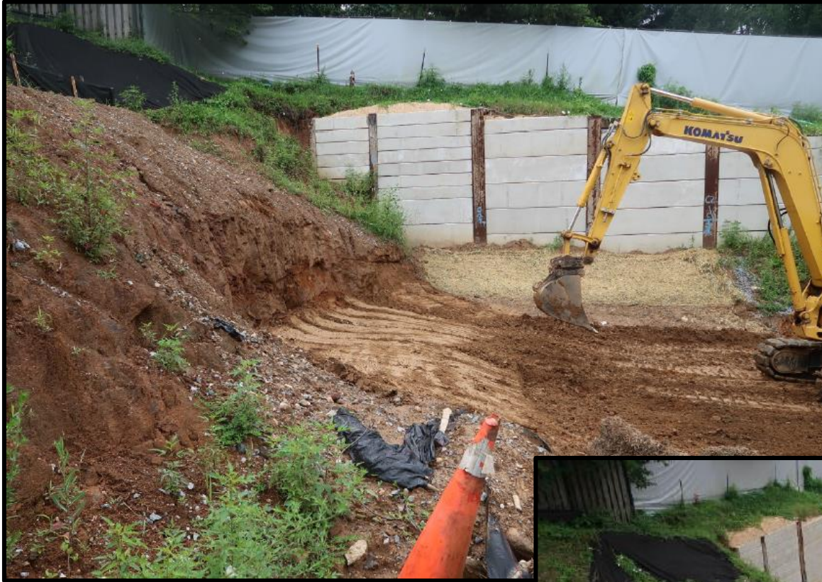
Backfilling grids with clean soil
