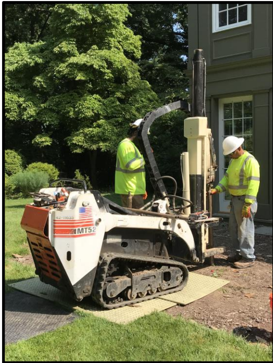
Collecting soil borings
