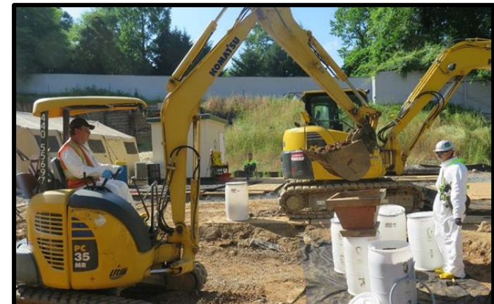
Mini-excavator placing soil into poly drums
