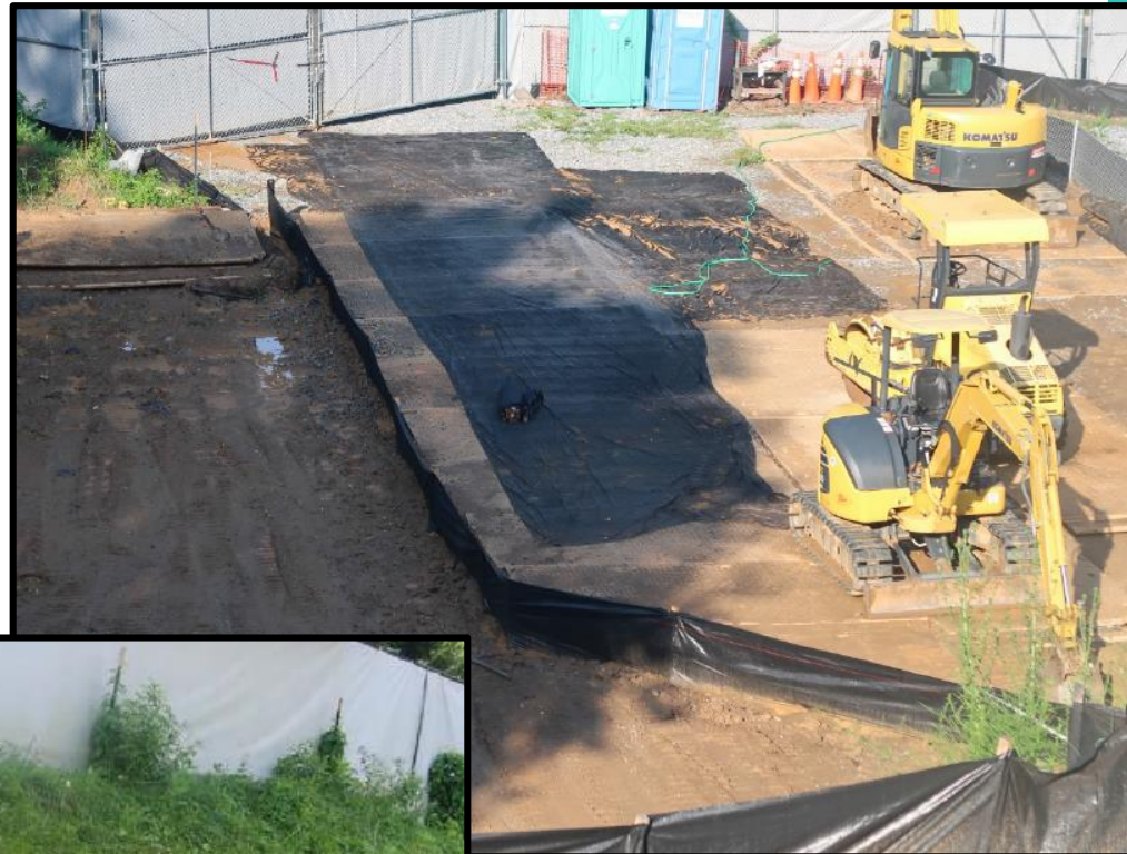
Erosion and Sediment Controls
