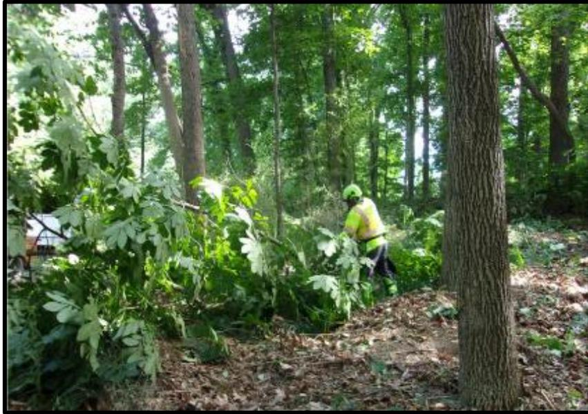
*Removing low underbrush and plants to achieve a clear line of sight between the robotic totaling station (RTS) and the survey equipment.*
