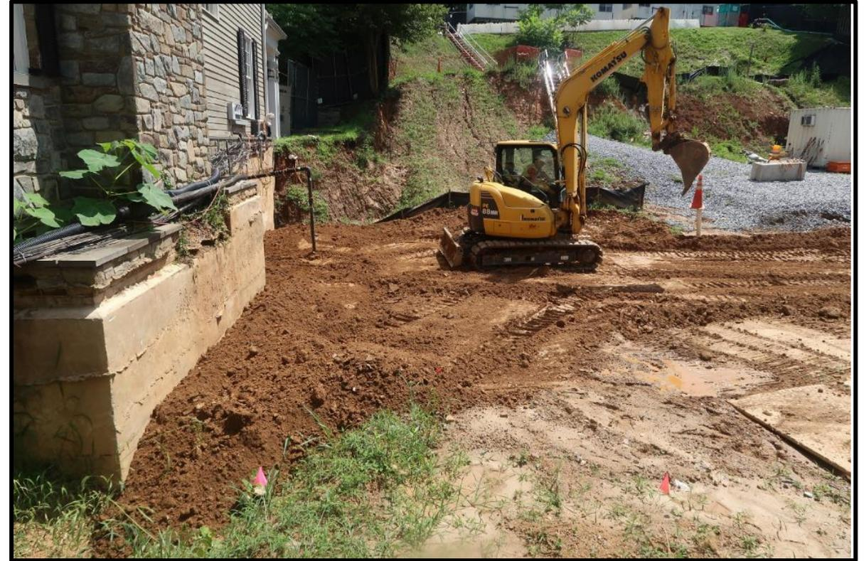
*Clean backfill along 4825-4835 property boundary to avoid water pooling near the foundation*
