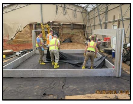
This included setting up an area designed for decontaminating large pieces like excavators, with a frame and liners that retained any water and soil cleaned off of equipment.
