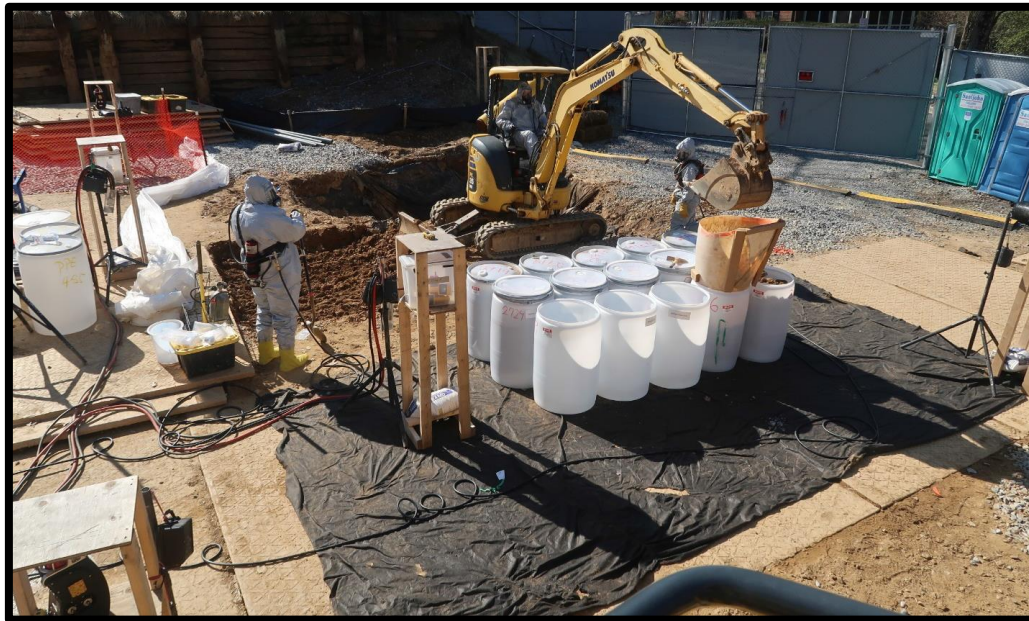
Area 4 Drum filling area with air monitors
