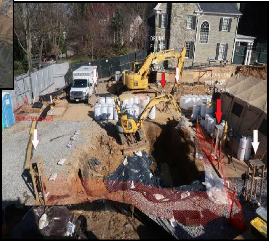
Area being excavated within Area 4 when MINICAMS alarms were triggered (looking southwest towards Glenbrook Rd.)
