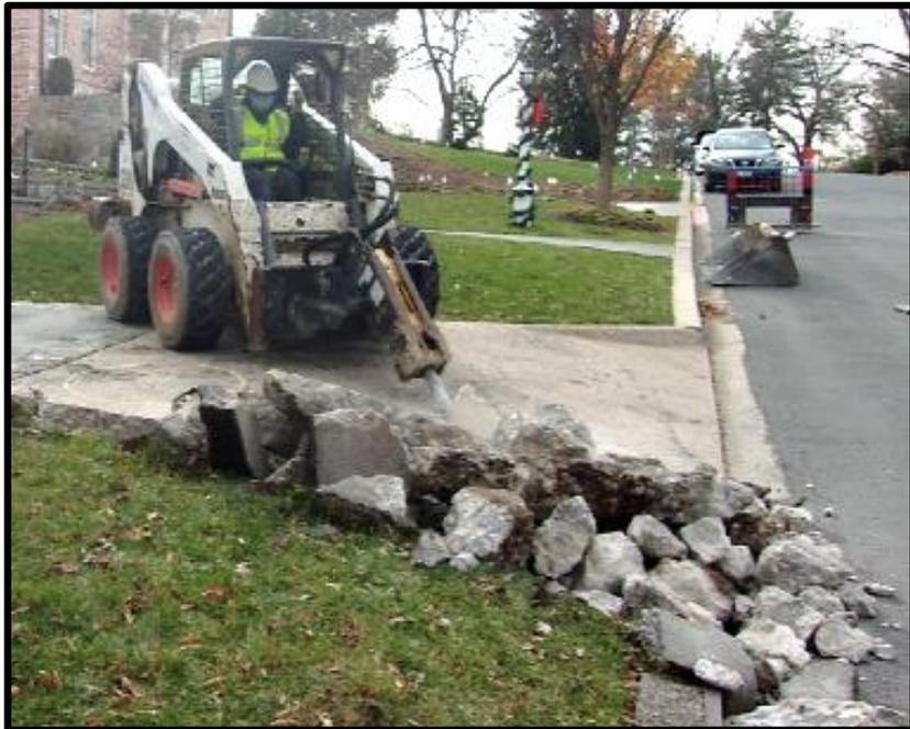
***Breaking up a concrete driveway apron to complete the investigation and removal of an anomaly under a driveway.***
