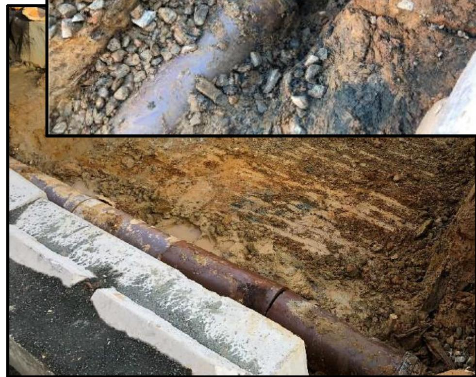
***Terra cotta pipe removed from Grid Cell F3***
