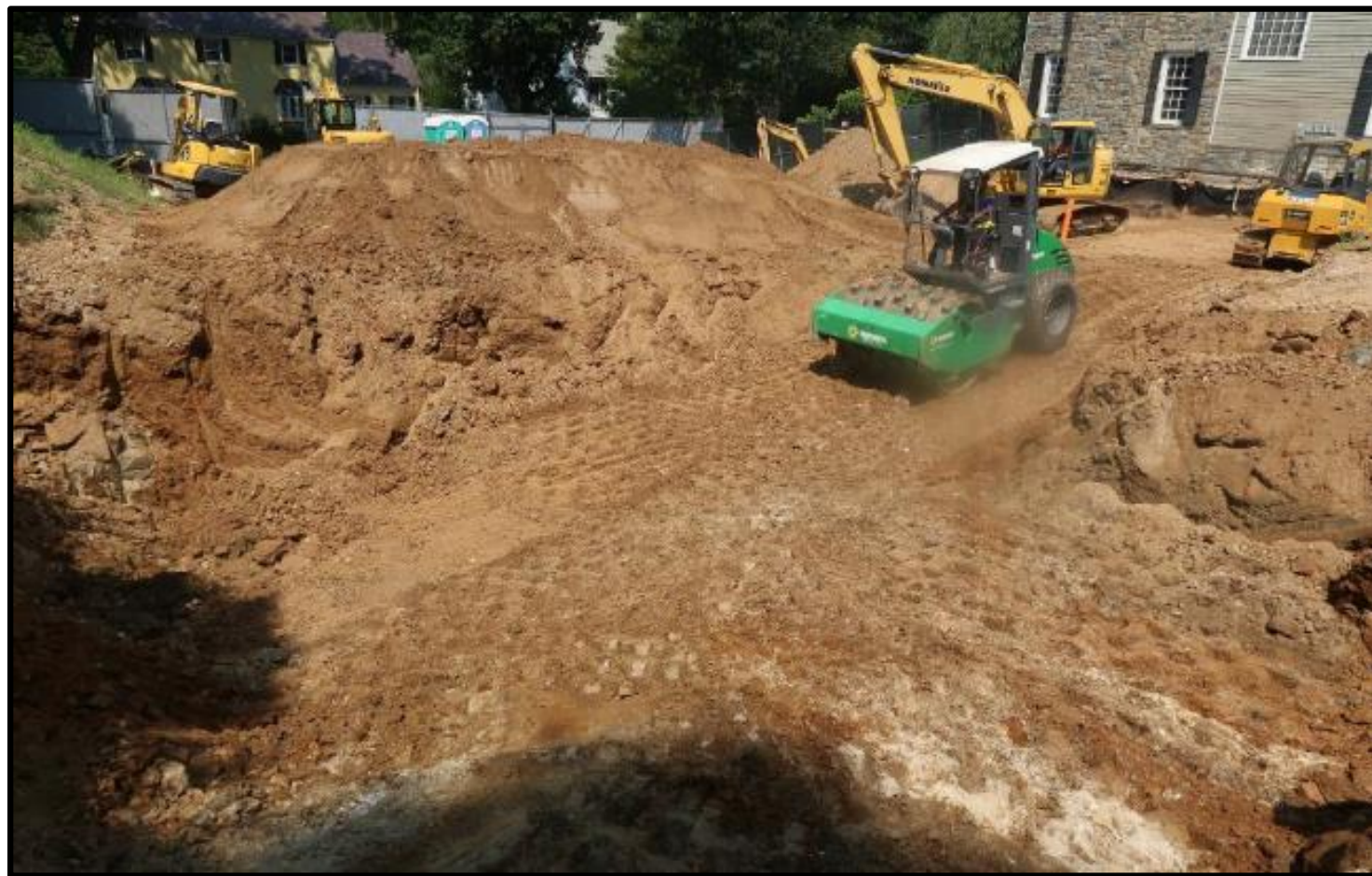
Compaction of clean backfill soil
