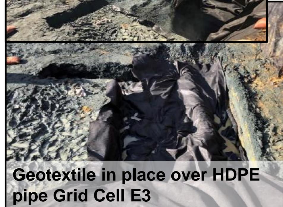
**Geotextile in place over HDPE pipe Grid Cell E3**
