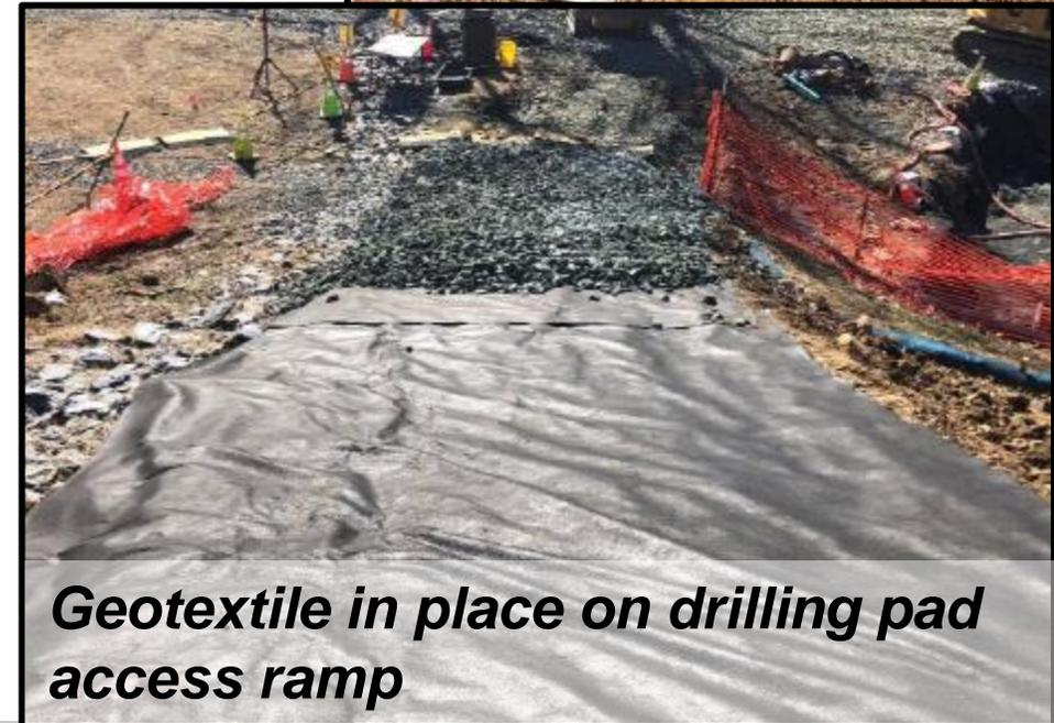
*Geotextile in place on drilling pad access ramp*
