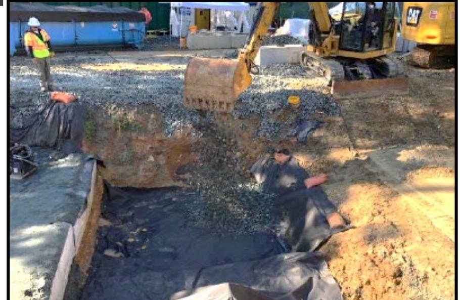
***No. 2 stone filled on top of geotextile during backfilling activities in Grid cell F5***
