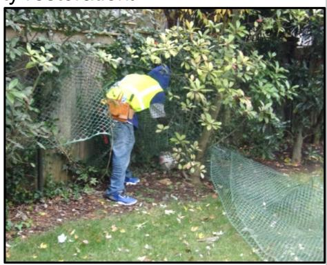
Removing temporary fence to install new fencing during site restoration.
