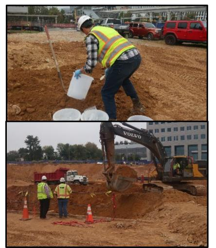
Sampling soil and inspecting a site for the needed backfill.
