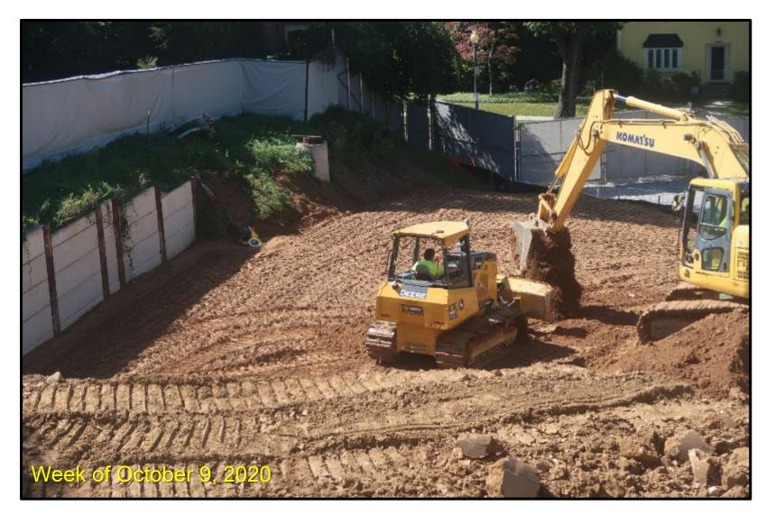
We have completed around 30% of the planned backfill and compaction effort to fully restore the site.
