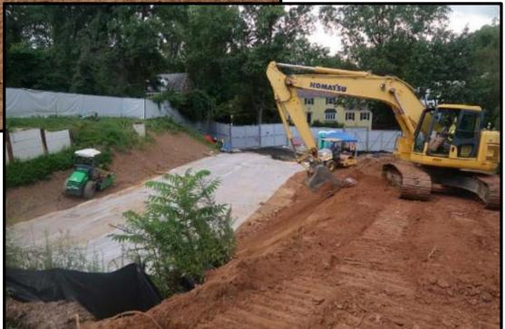
Backfill efforts are currently being conducted at the south end of the property, per a planned standard construction-grade approach. We currently are at around 30% complete with the backfill and compaction efforts at the site.
