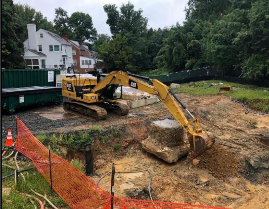
Excavator preparing to roll the concrete sump structure out of the excavation for sizing.
