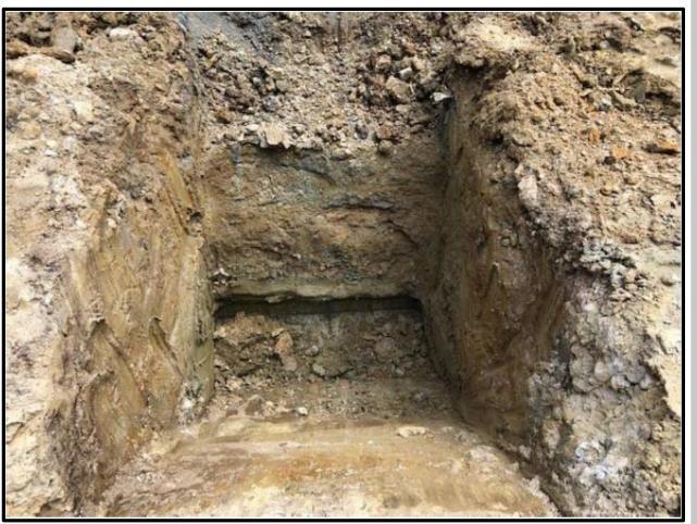
Test pit in Grid E-4 excavated to 8 feet below slab grade
