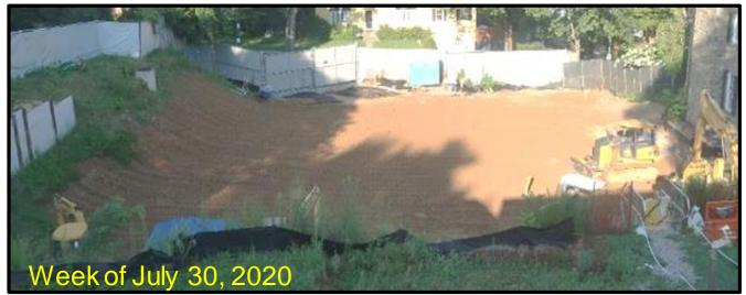
As the crew completed backfilling the small excavation areas, the focus moved to restoring the site's planned elevation, compacting to street level during the week of August 7<sup>th</sup>. Then operations continued on the south side. The compaction efforts involve close monitoring and inspection of the moisture
