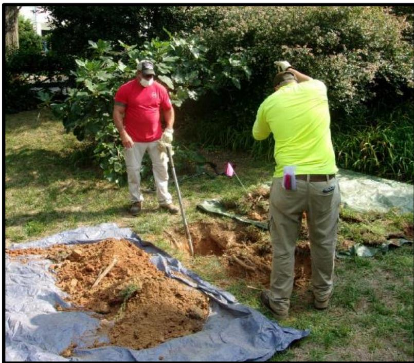
The team carefully excavates each area on the dig list. Grass and soil are placed face down on a tarp, to be seamlessly replaced after removing anomalies.
