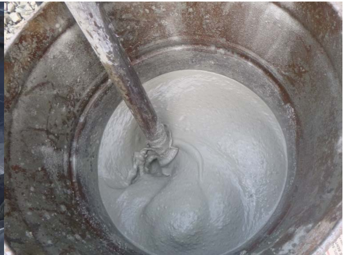
Mixing grout to abandon bore holes
