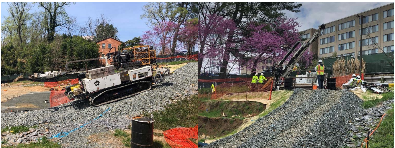
Track-mounted roto-sonic drill rig on ramp
