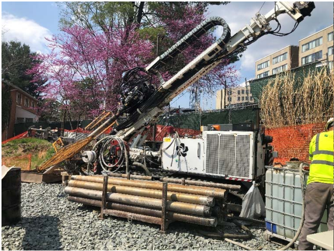
Rosonic drill rig set up for angled boring
