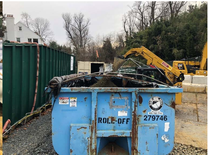
Processed soil being loaded into roll-off container for disposal
