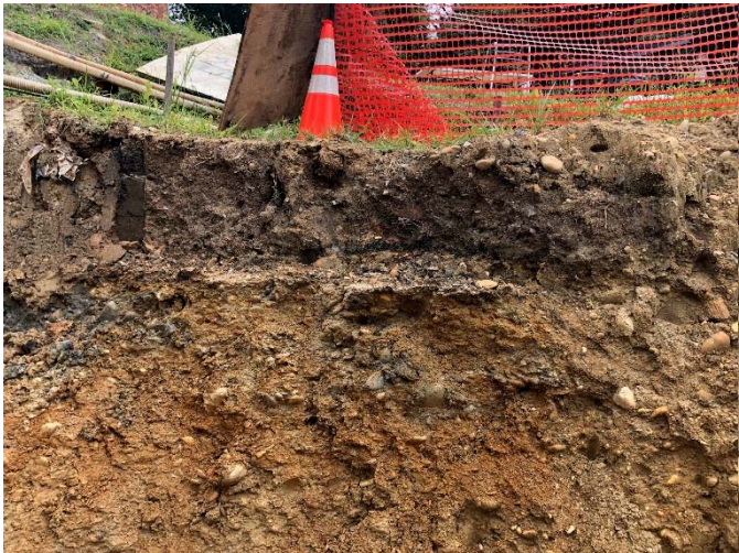
Impacted soil layer in PSB eastern sidewall, north end, at sanitary sump
