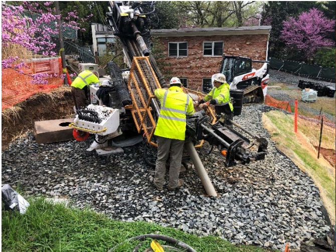
Drilling crew set up for roto-sonic boring
