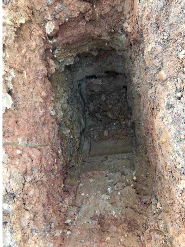
Test Pit E8 Excavated to 9 ft
