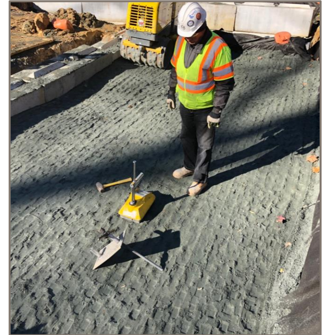
Density Testing – Using Troxler nuclear density gauge to test compaction.
