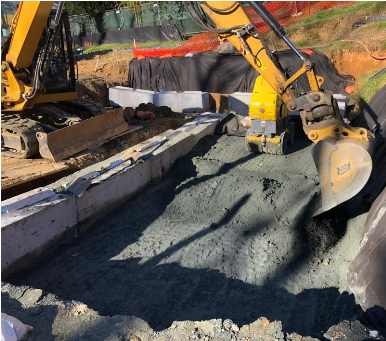
PSB Operations – Crushed rock backfill from Aggtrans Savage Quarry, Jessup, MD being placed in excavation.
