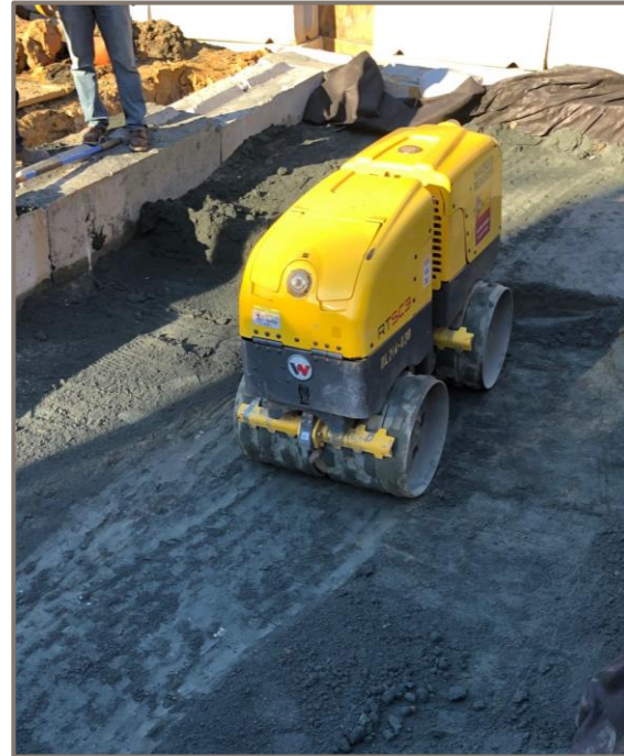
Compaction – Using Vibratory drum trench compactor.
