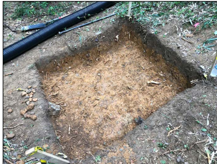
Completed RA1 excavation at 5 ft by 5 ft by 1 ft deep.
