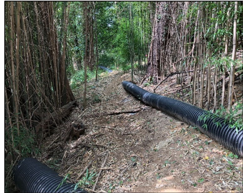
Access path to RA1 through bamboo from RA2 location with AU drain lines.
