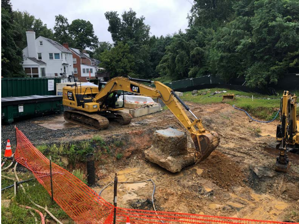
PSB Operations – Excavator moving the sanitary sump and footer prior to breaking it up for disposal.
