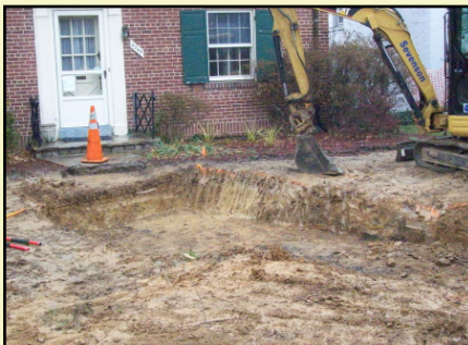
Photos showing the arsenic removal work completed at a residence in Spring Valley in 2008 and the same property after it was restored following the removal action.
