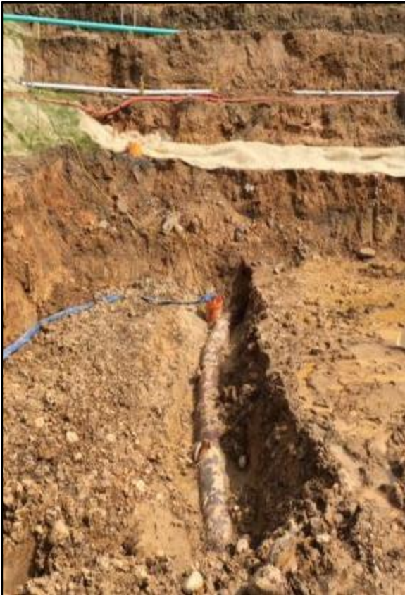
Terracotta Pipe along the edge of Grids E2 and F2 at 5 feet bgs
