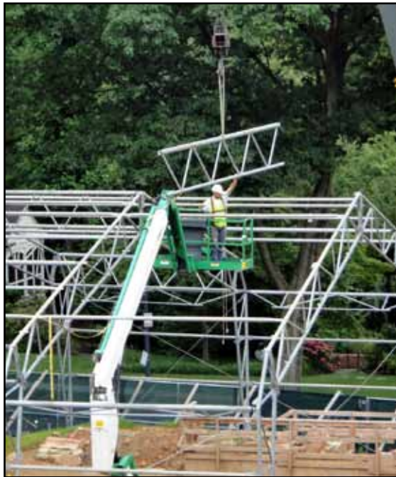
Construction of the Engineering Control Structure
