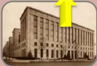
Bureau of Engraving & Printing Advise, design and construct new printing facility in Beltsville, MD
