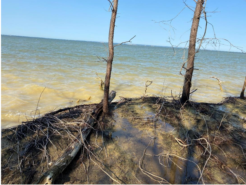
9) Shoreline on western portion of island, facing west
